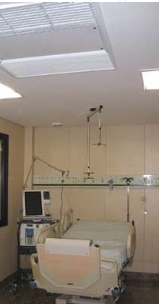
Hospital Mater Dei, Belo Horizonte (MG)
