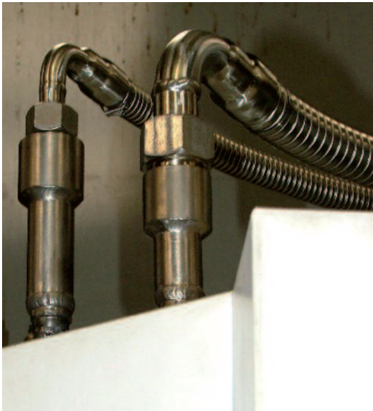
Flow/return connections to CO 2 OLrac
