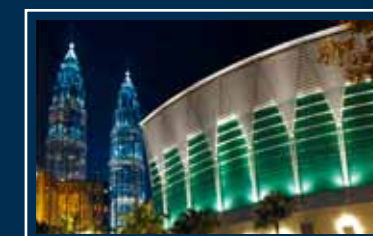
Kuala Lumpur Convention Centre, Malaysia
